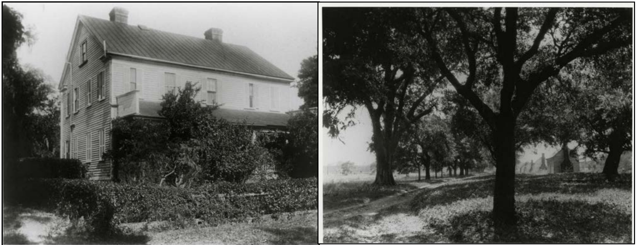
Figure 18: McLeod house and cabins, c. 1930 (Photos by William Henry Johnson, collections of the South Carolina Historical Society).
