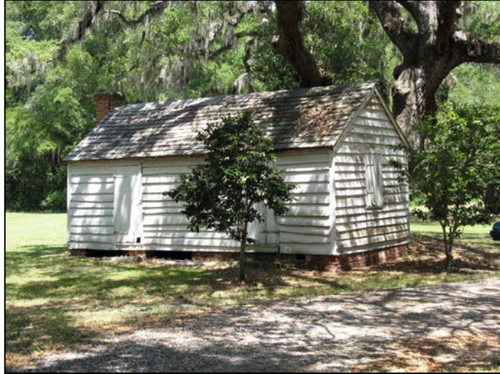
Figure 66a,b: Views of the dairy; a) facing northwest. The cellar foundation is visible on the right side of the structure, b) position of live oak relative to north side of the structure.
